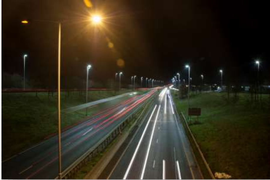
LED Improvement Project
