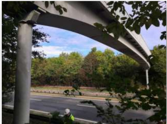
APV Baker Footbridge
