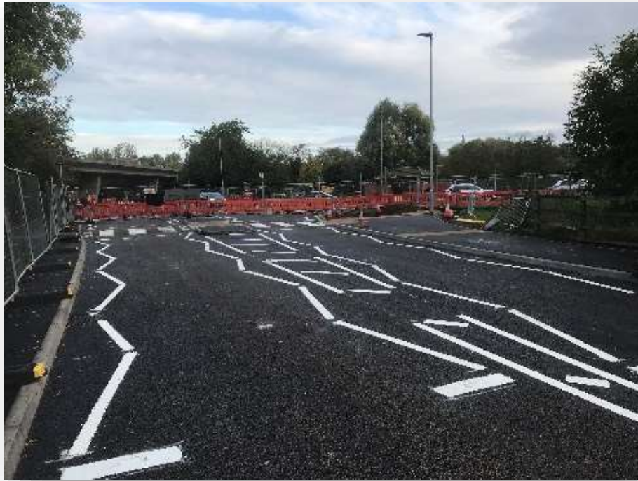
Whittlesey Road Pedestrian Crossing
